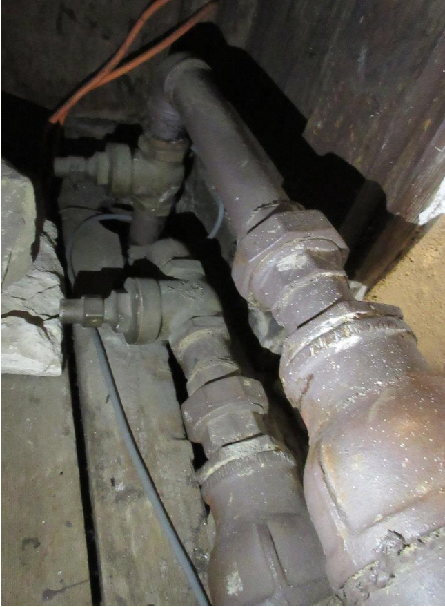
The existing valves within the North Aisle.
